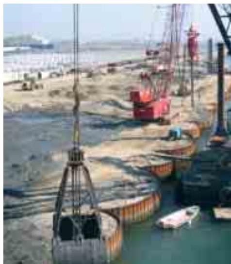
strong potential for liquefaction at depths of up to 18 m. The effects of soil liquefaction include loss of foundation bearing capacity and side friction capacity, surface settlements and risks of circular slips in submarine slopes adjacent to the sheet pile curtain.
