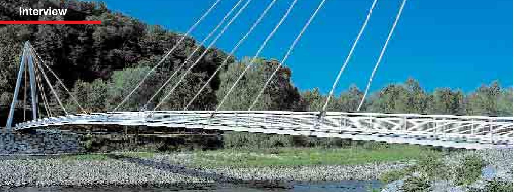
Carbon fibre cables, installed on the Laroin footbridge in France, contribute to improving the durability of structures.
