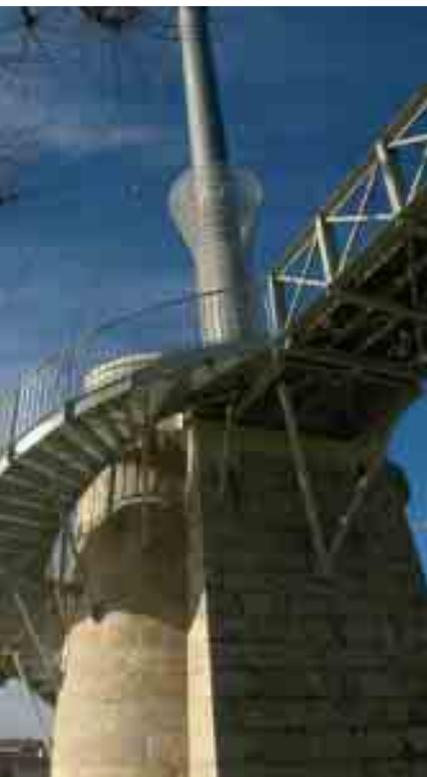
The solution proposed by Freyssinet consists of replacing the suspension, and the tower and deck cable anchors. This is a seventeen-month project.
